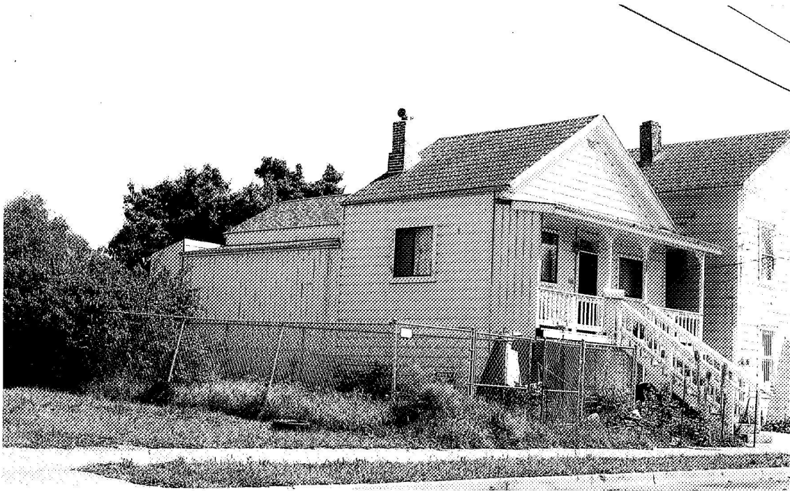
Figure 4. Worker's cottage on Chester Street, West Oakland, begun c. 1875. Starter cottage at the front (right), with several later additions to the rear (photograph by the author, 1995).
