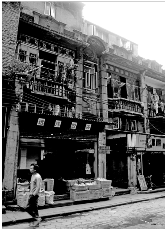
Figure 9. Zhutongwu apartment building, 29 Baoxiang Nanlu, Guangzhou (authors' photograph, 2007).
