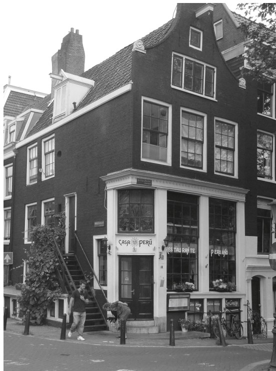
Figure 13. Façade of a commercial-residential building in Amsterdam. Even though the windows on the front façade serving residential space are large, there is still a strong distinction between that part of the façade and the shopfront below. This illustration also shows at least two separate entrances to residential parts of the building. Photograph by the author.
