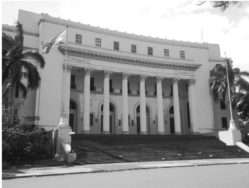
Figure 6. Museum of the Filipino People, a building formerly known as the Department of Finance. Located on a site close to where Burnham was to place the Capitol Building, this building was to form an integral part of Manila's civic core (photograph by the author, May 2010).
