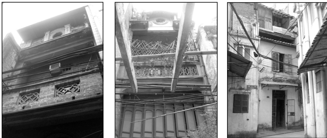
(c) Photographs of the mixture of material on façades of multi-family zhutongwus .
