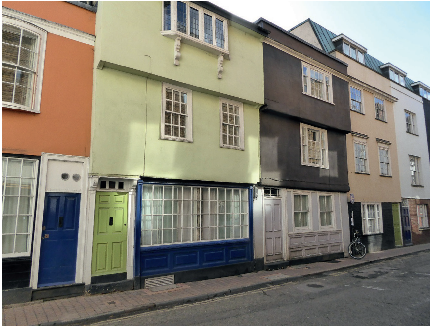
Figure 2. Street façade Pembroke Street.
