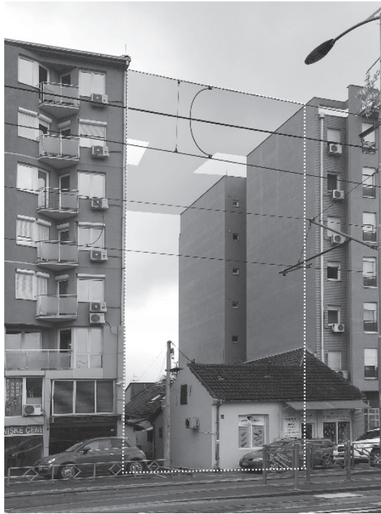
Figure 2. Street frontage: the old and the new.
